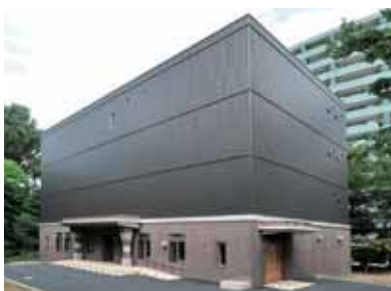
Specimen storage building for the Botanical Garden of the Field Science Center for Northern Biosphere
