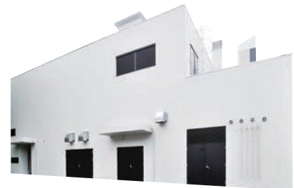
Chemical exposure and infectious disease experiment facility ■ Total floor area: 660 m 2 ■ Structure and No. of floors: 2-story reinforced concrete structure
