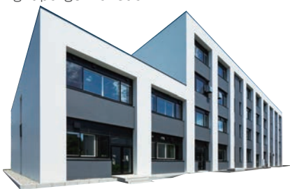
Civil Engineering Research Building ■ Building area: 1,385 m 2 ■ Total floor area: 4,392 m 2 ■ Structure and No. of floors: 4-story reinforced concrete structure
