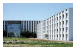
ICReDD Building New building design in FY 2020 - 2021 Energy saving 55% Equivalent to ZEB Ready
